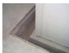
Excavation sample Dettaglio scavo
