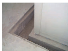
Excavation sample Dettaglio scavo
