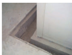
Excavation sample Dettaglio scavo
